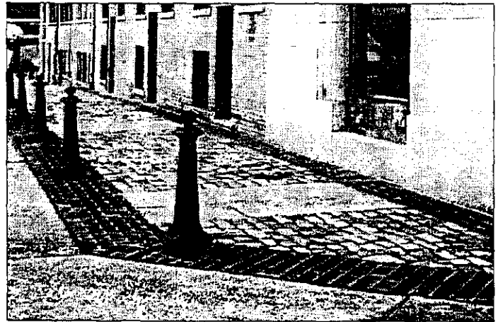
Features, such as brick sidewalks and decorative paving materials, like this sidewalk in Asheville, North Carolina, add character to a district and should be preserved.
